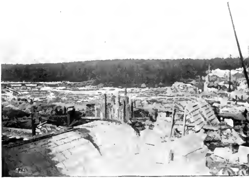
FIG. 5.—BUILDING THE DAM, GARVIN'S FALLS.
